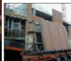
Delivery to site
